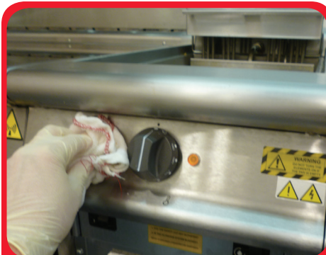
Step 8 - Wipe external areas, such as hob, hob front and door with a damp cloth.
